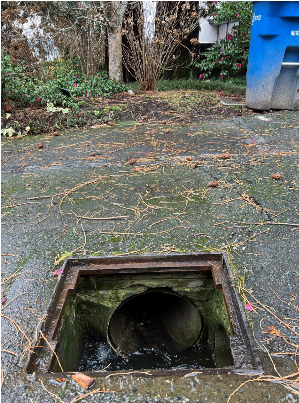
Photo 6: Catchbasin 18C-163 (looking west towards discharge point)
